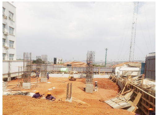
Foundation works; backfilling of the raft base and stub columns
